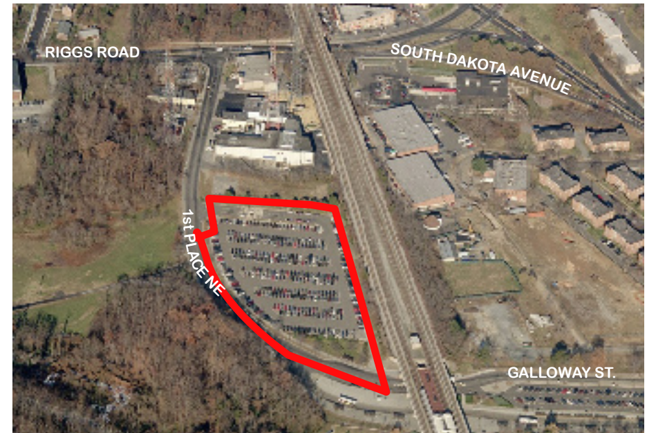
Figure 3.18 - Aerial of the Fort Totten West Parking lot
