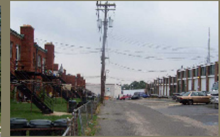
Conflicting land uses - residential across the alley from industrial land uses at 2nd Street
