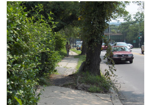
Figure 2.18 - Non accessible sidewalk on Riggs Rd
