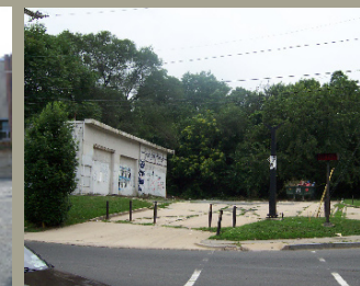
Abandoned gas station at 1st Place
