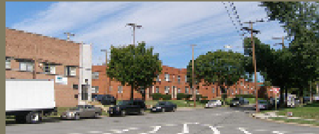
Conflicting land uses - residential abutted to industrial land uses at 3rd Street
